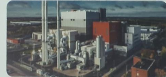
Implementation of huge biofuel CHP 170MW in Vilnius
